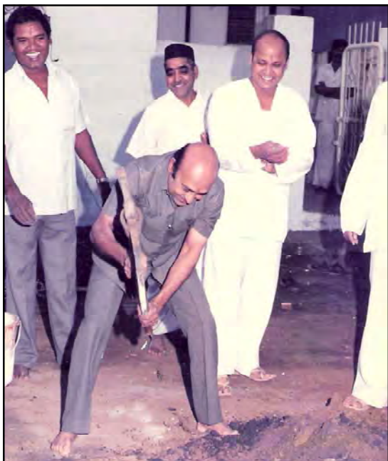
(Punambhai commences the digging for plinth of the Pavilion)
