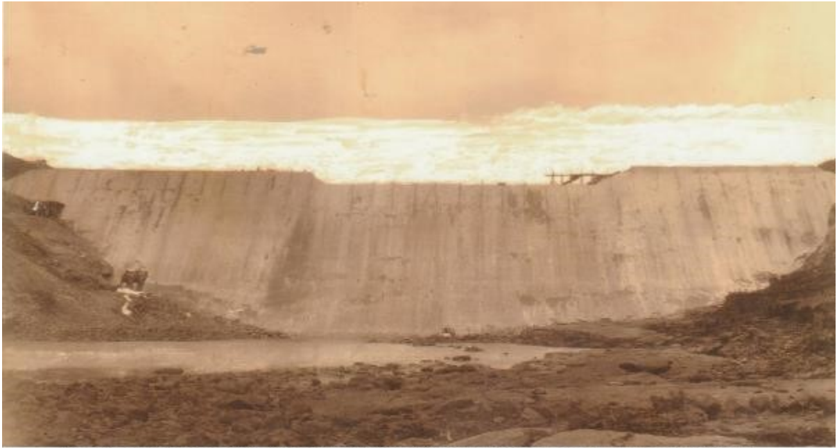
58 - Dam in May 1918 Average height 135 Ft. Above River Bed Down Stream face from River Bed
