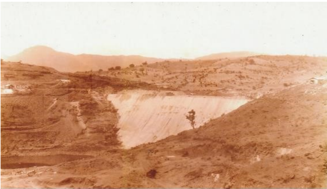
65 - Dam in May 1919 Effective Height 155 Ft. Above River Bed Down Stream face from the North Bank.
