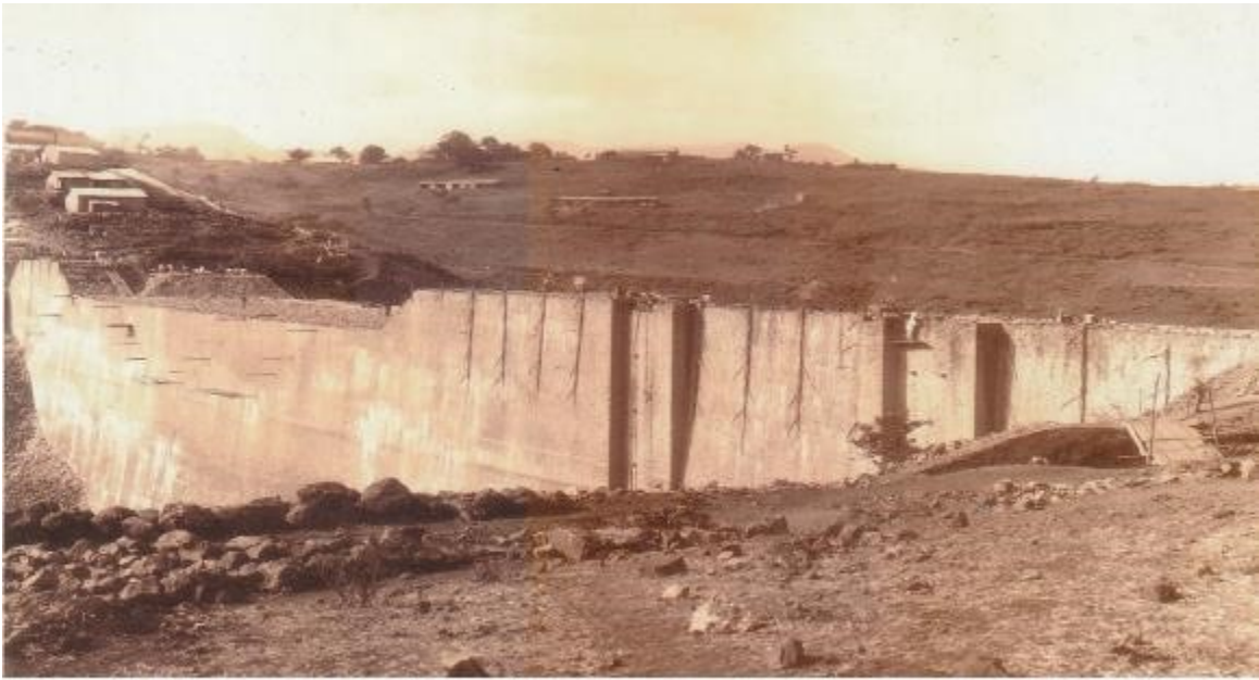
66 - Lake Aurther Hill Dam - Full View of the DAM 155 Ft. High ( June - 1919 ) Up Stream face from the South Bank.
