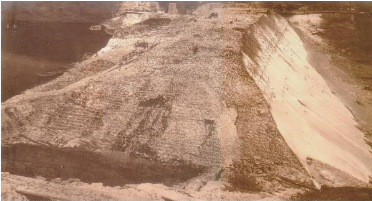
52 - Dam in May 1917 Average Height 113.25 Throughout Down Stream Face from River Bed
