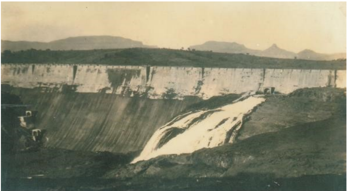
45 - Down Stream View with 200 Ft. Sluice Open
