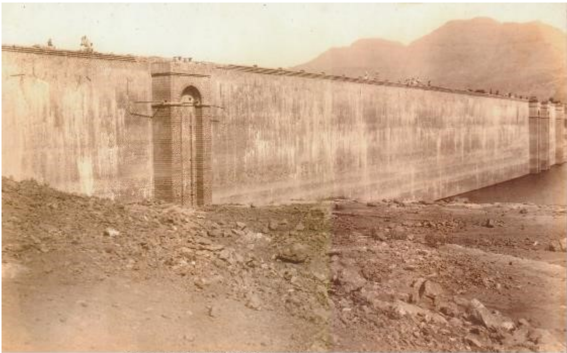
21 - Dam in May 1924 Height Ft. Up Stream View from South Bank
