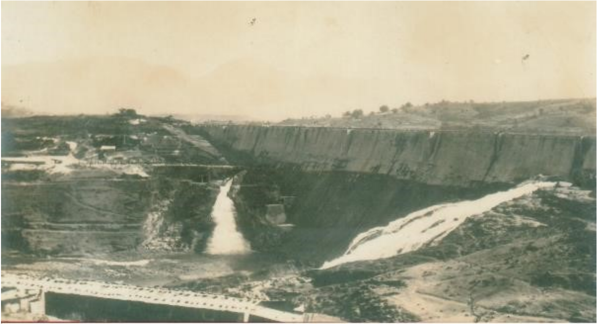
44 - Down Stream View with 150 a 200 Ft Sluice Open
