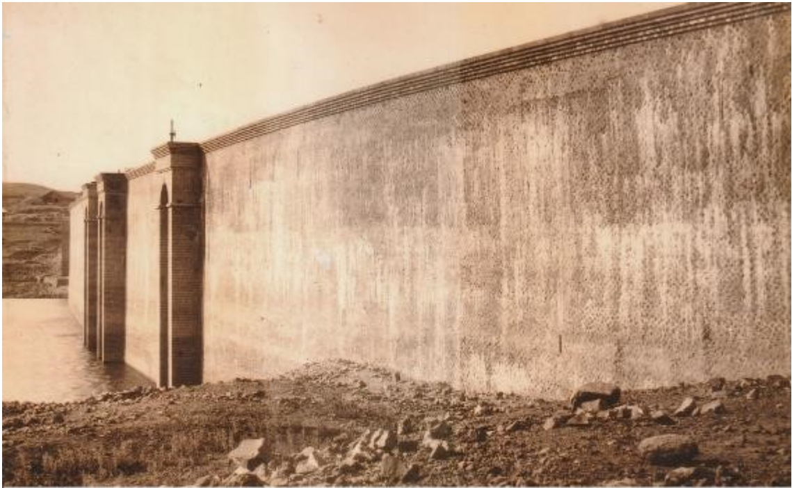
20 - Dam in May 1924, Height 270 Ft. above River Bed . Up Stream View from North Bank
