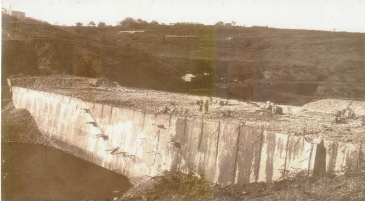
56 - Dam in May 1917 Average Height 113.25 Throughout Down Stream face from the South Bank
