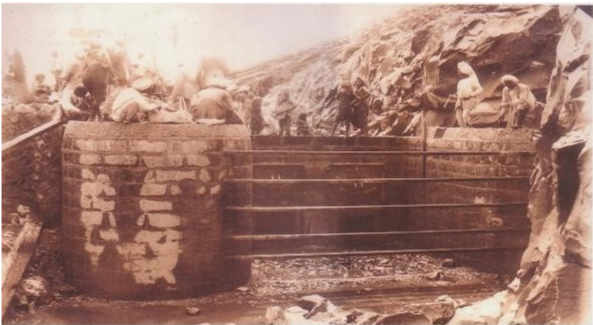
57 - The Second Set of the Steel Outlet Pipes at 100Ft. Above River Bed in Progress Showing Casing Arrangement ( May - 1917)
