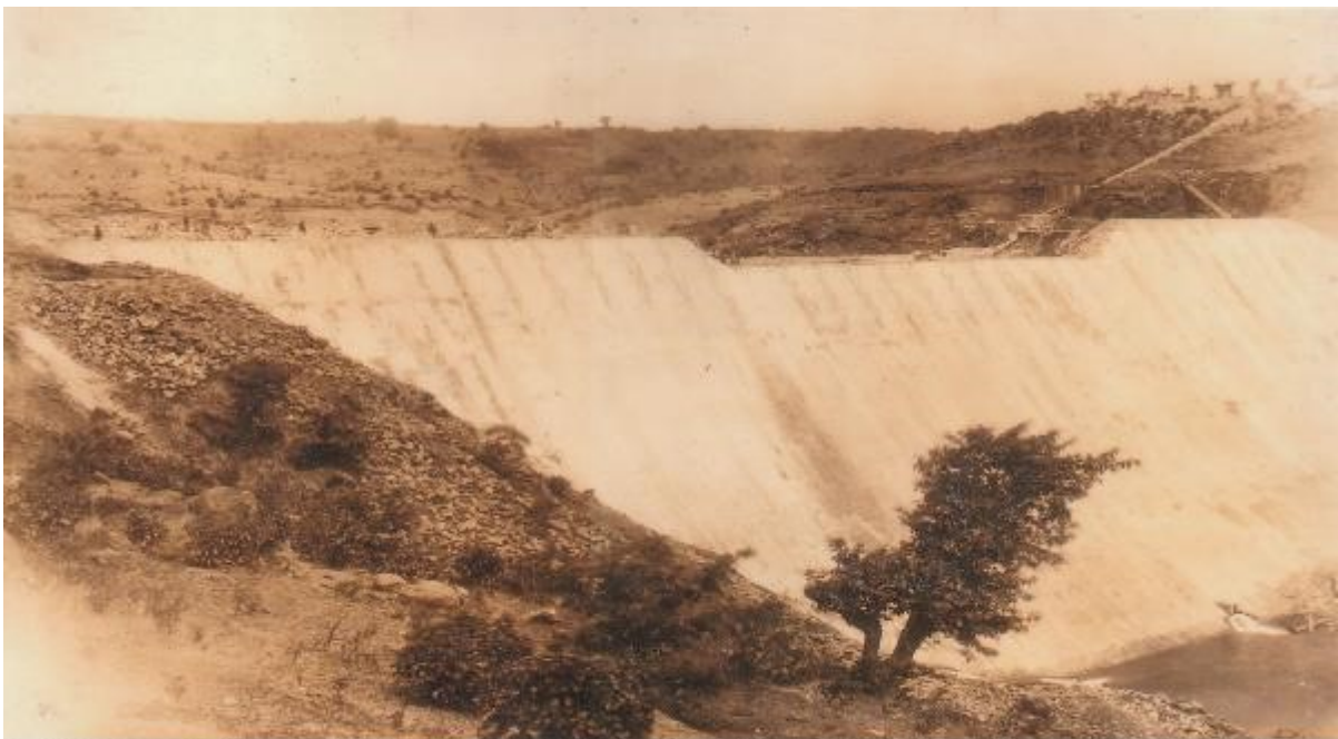
59 - Dam in May 1918 Average Height Ft. Above River Bed Down Stream face from the South Bank
