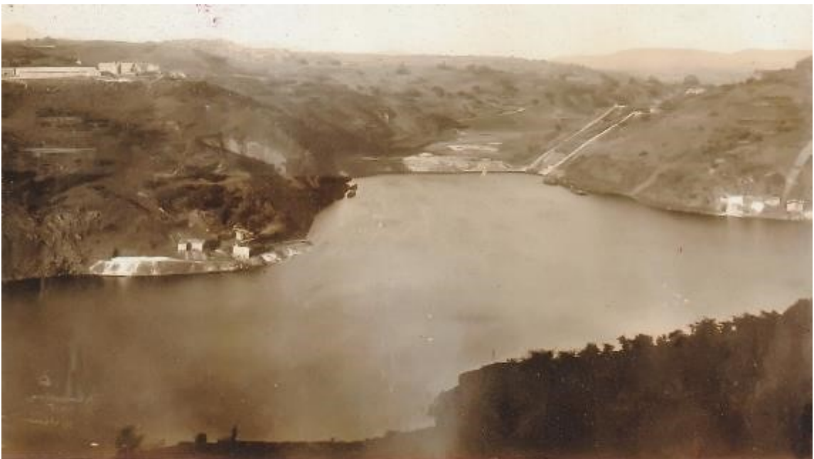
15 - General View of the Dam - 1915.
