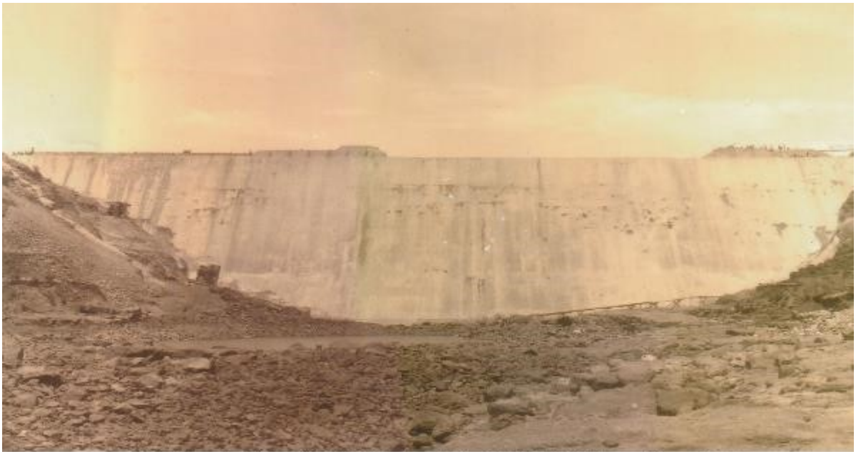
64 - Dam in May 1919, Effective Height 155 Ft. Above River Bed Down Stream Face from River Bed.
