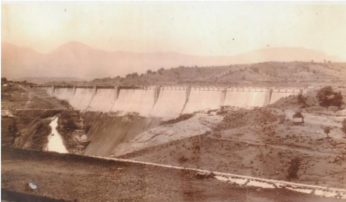
18 - General View of the Dam .May 1924 Height 270 Ft Showing 35 Arches Completed . Down Stream View from Cause - Way Bellow Dam
