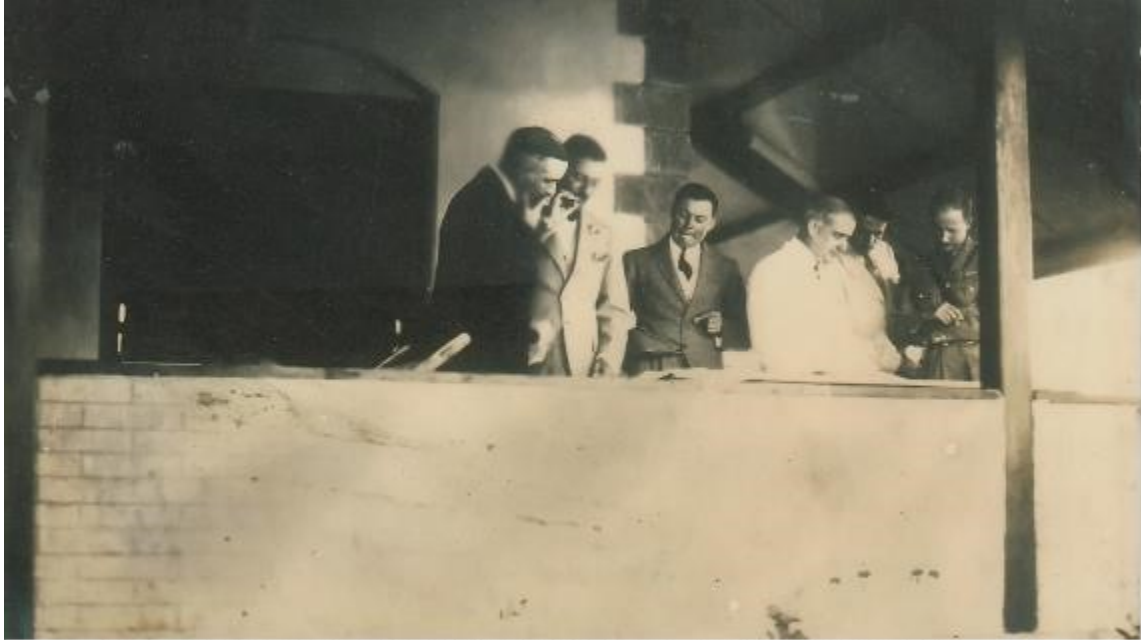
33 - Suoerintending Engineer, Deccan Irrigation Division, Explaining, His Excellency the Working of Hydralic Ramp.
