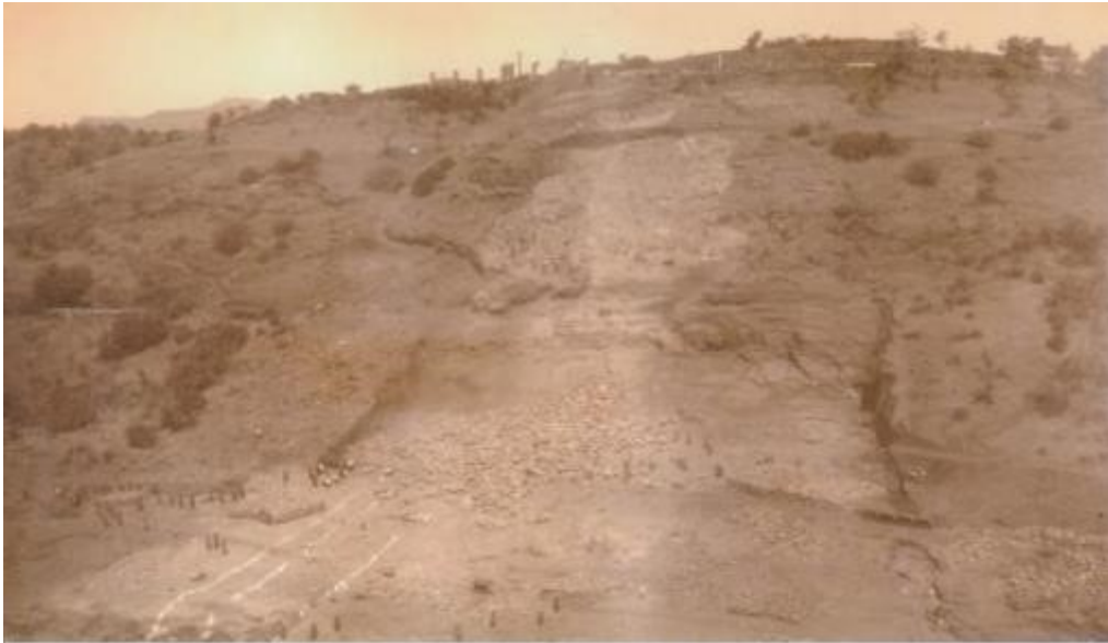
2 - Lake Arthur Hill Dam - Clearing Foundation , 1912
