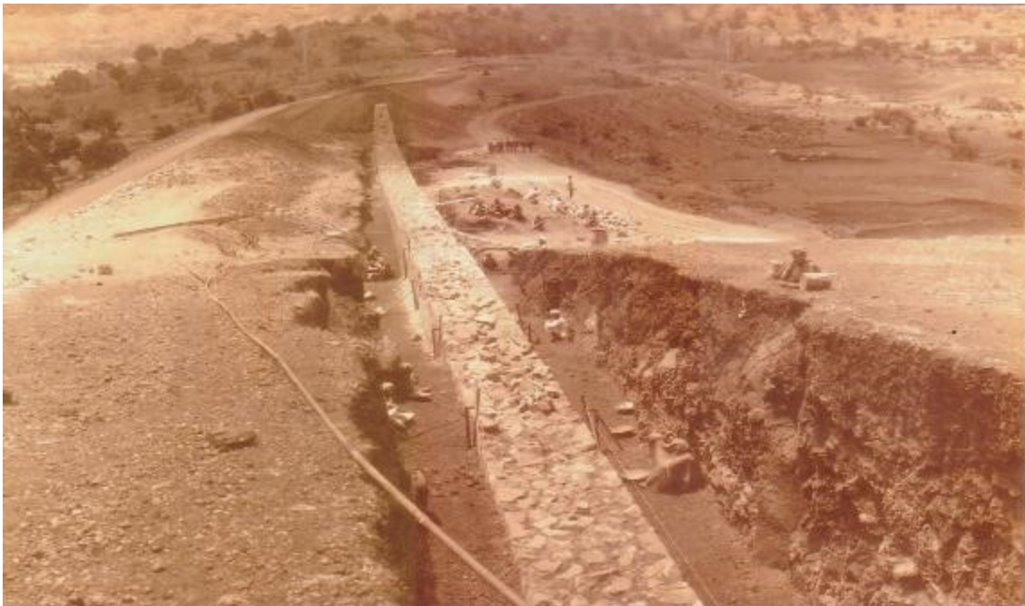
73 - Embankment Over the Low Saddle Showing the Masonry Core Well - 1919
