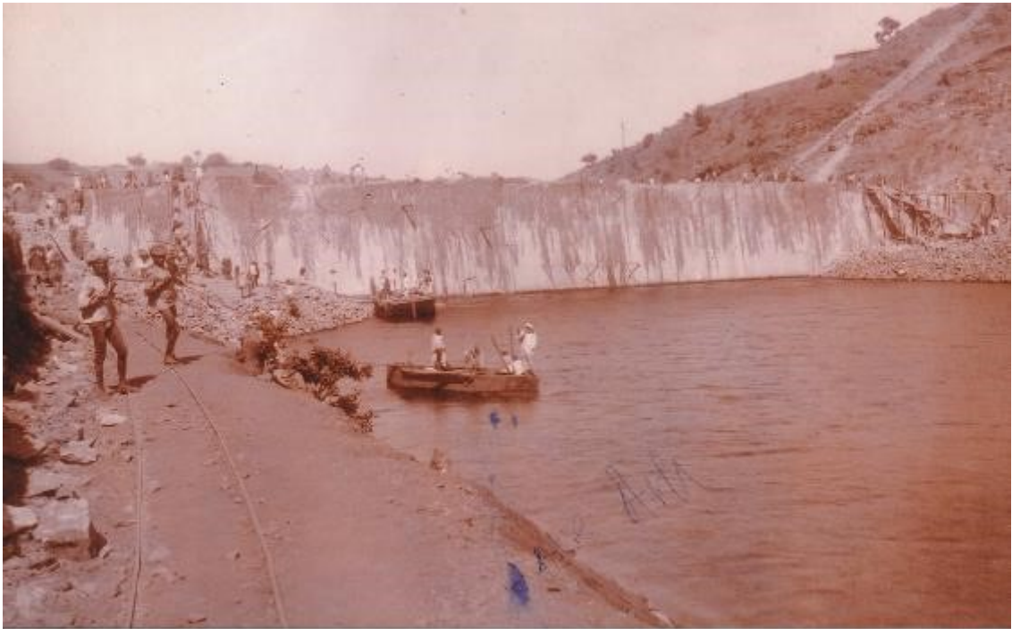
10 - Lake Arthur Hill Dam - June . 1914 , 70 Feet High Up Stream.
