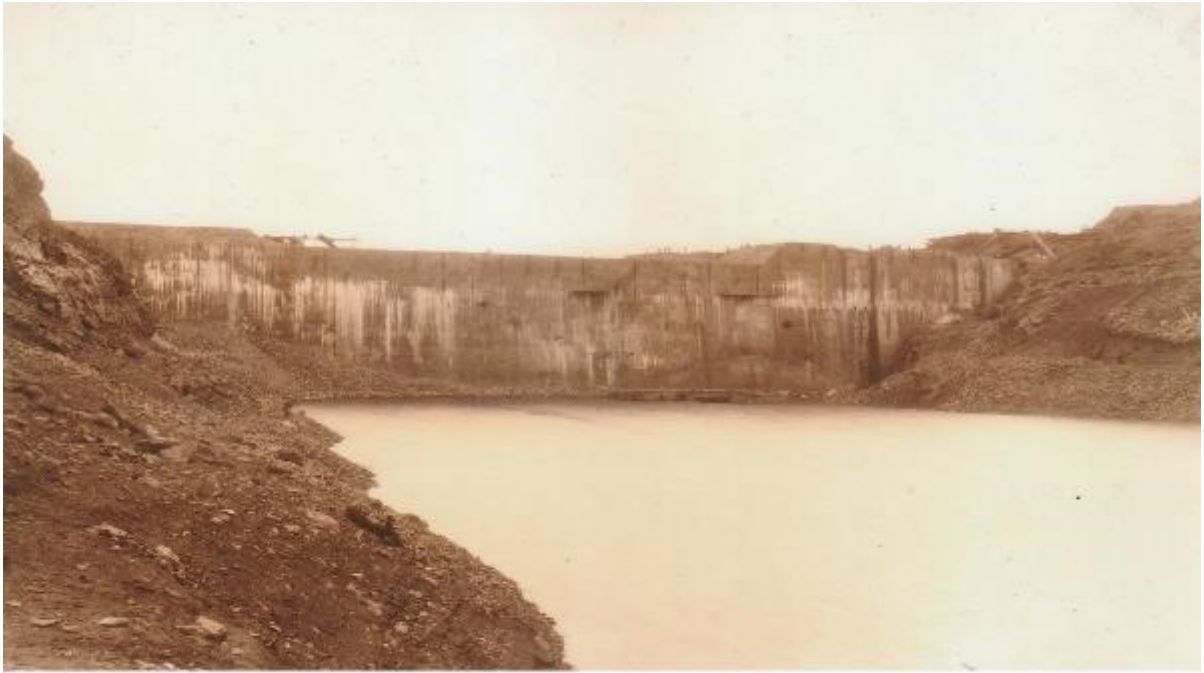
62 - Dam in May 1918 Average Height 135 Ft, Above River Bed Up Stream Face From The South Bank ( Full View of the Dam )
