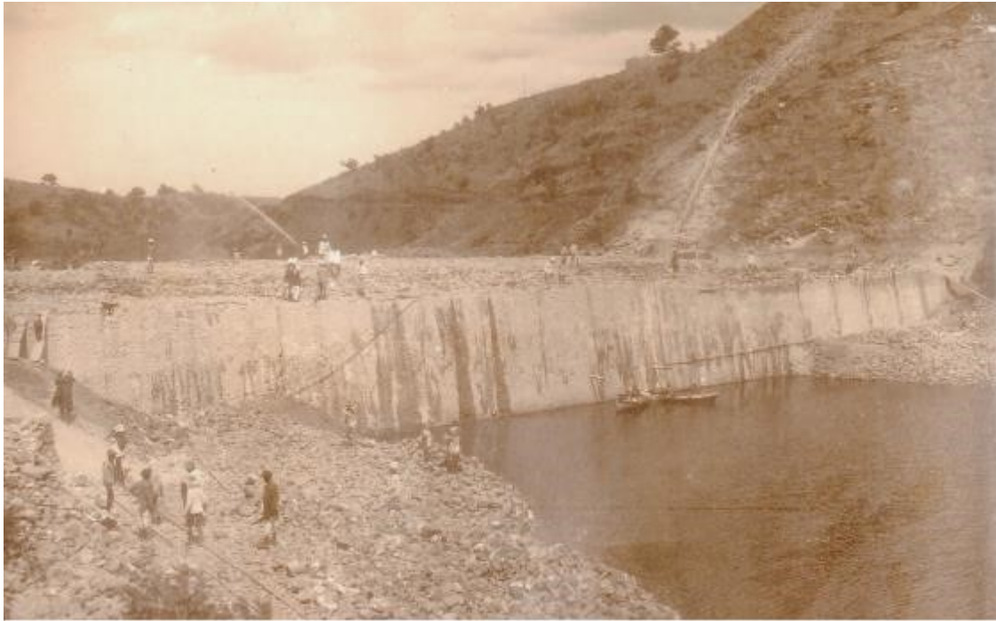
6 - Up Stram View of the Dam from Left Bank ( Never View ) - June , 1913
