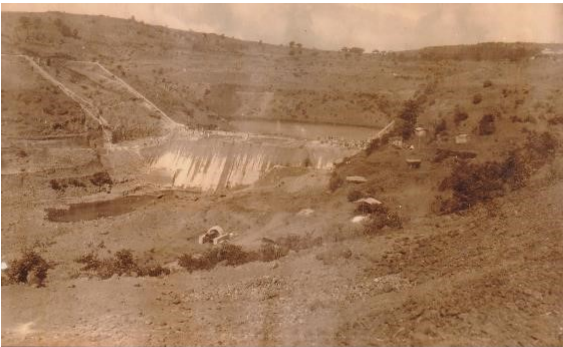
9 - Lake Aurthor Hill Dam - Full View of the Dam taken from the Left Bank Down Stream ( June - 1914)
