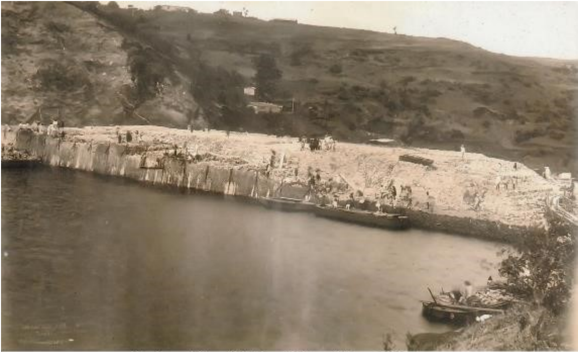
14 - General View of the Dam Up Stram ( June - 1915)
