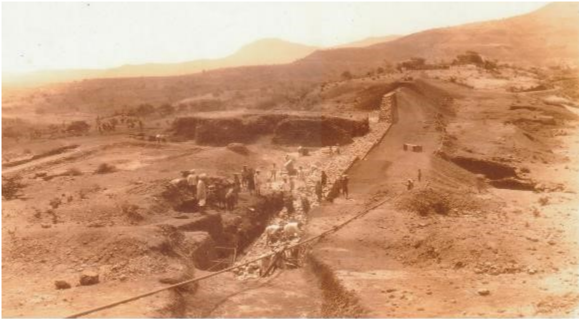
74 - Embankment Over Abandoned Waste Weir Showing Masonry Core Wall - 1919
