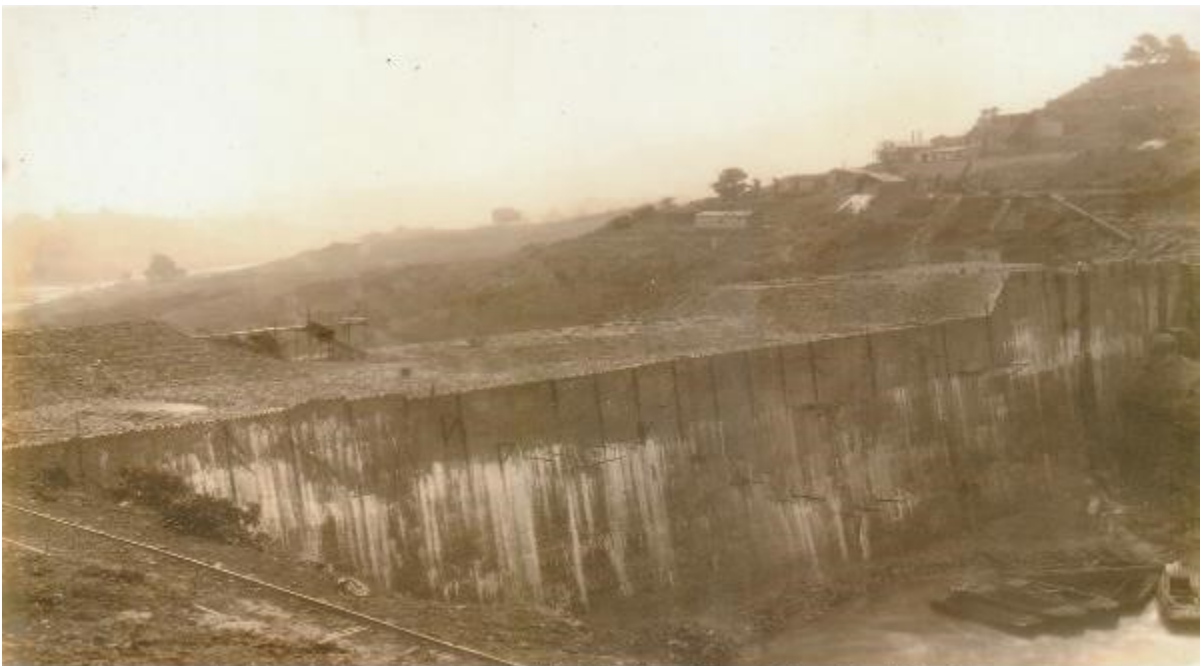
61 - Dam in May 1918 Average Height 135 Ft. Above River Bed Up Stream Face from the North Bank
