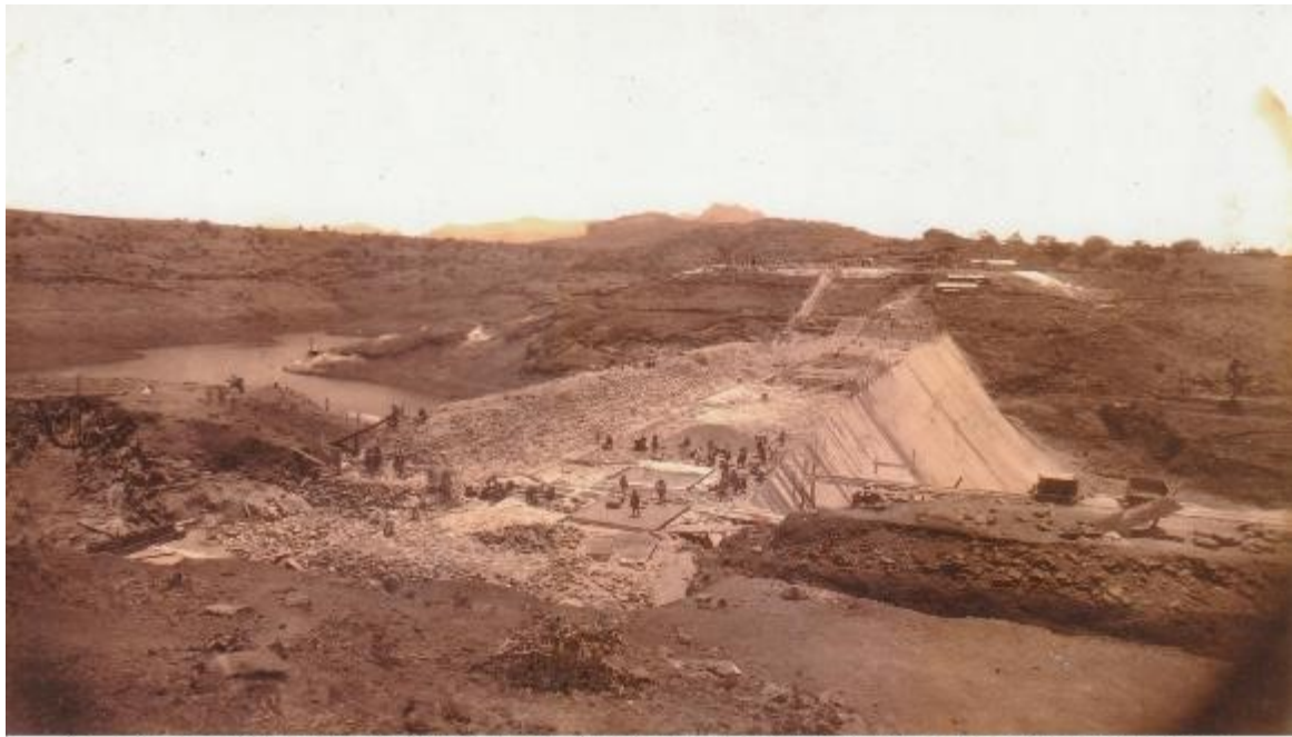
68 - Dam in May 1919 Effective Height 155 Ft. Above River Bed Top View of the Dam ( Nearer View)
