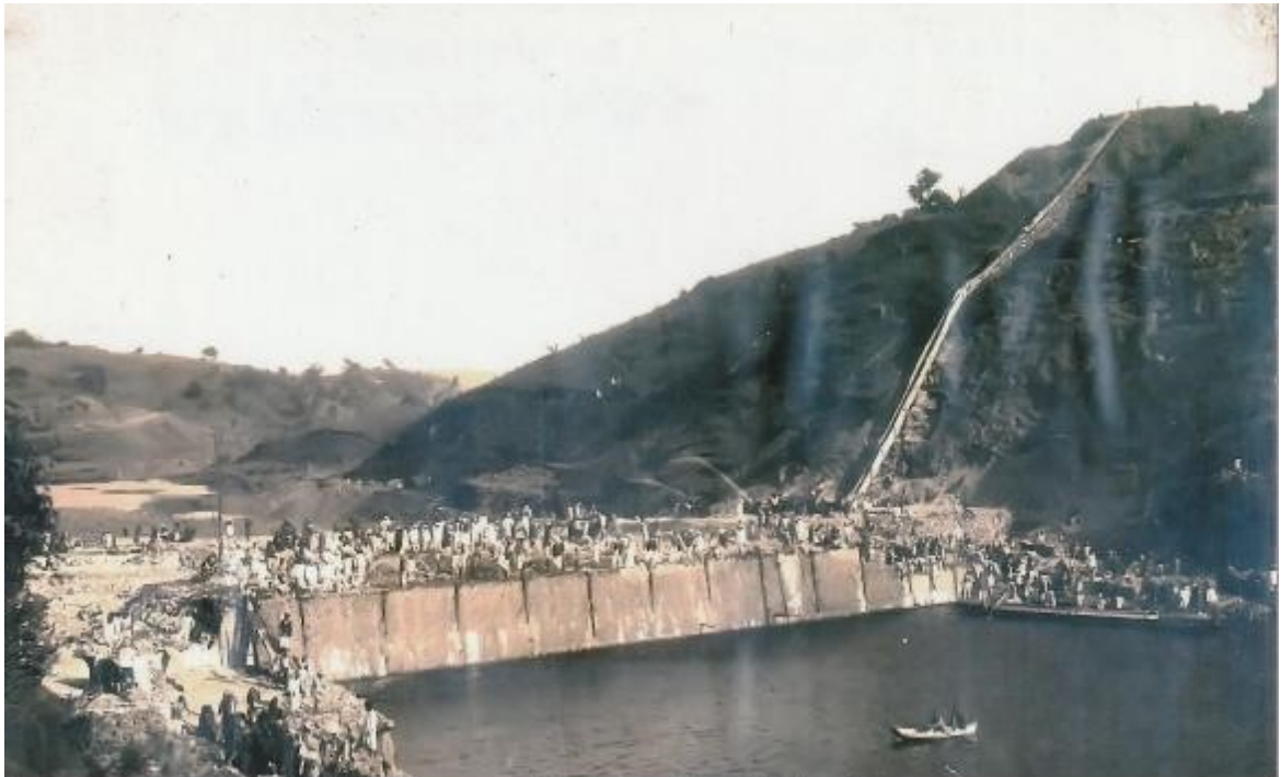
Almost all the Labourers on Bandardara Dam Construction.
