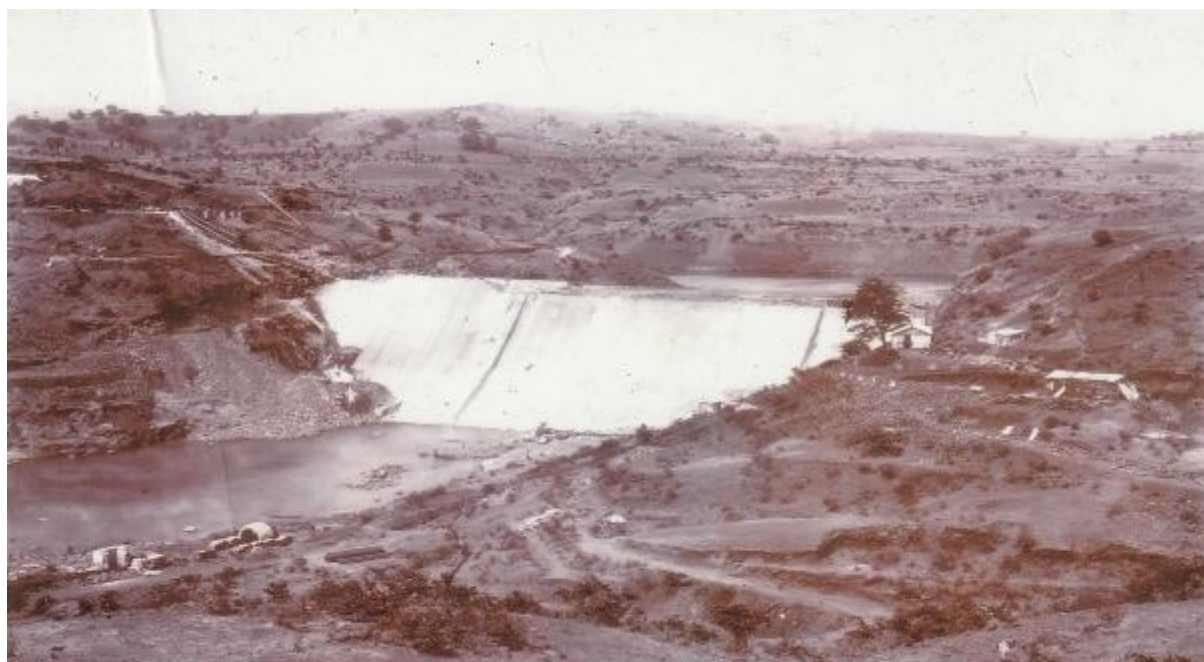
55 - Dam in May 1917 Average Height 113.25 Throughout Up face from the South Bank
