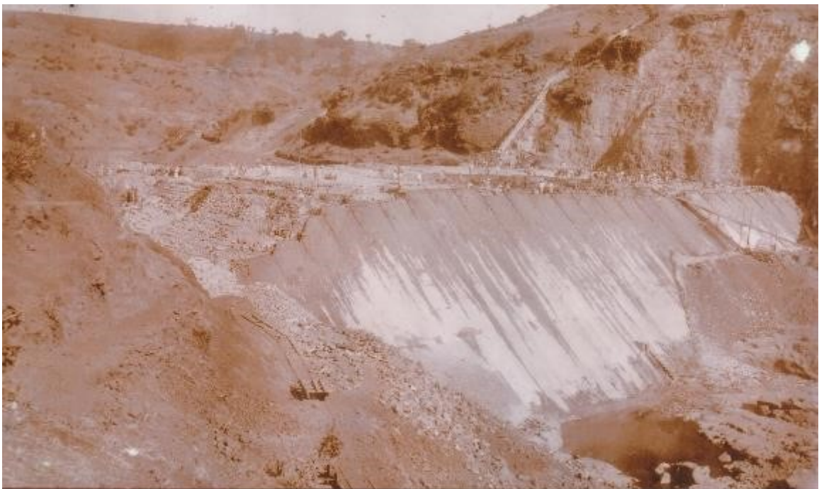
11 - Dam in June 1914 . Effective Hight 70 Ft. Above River Bed top View of the Dam from Down Stream
