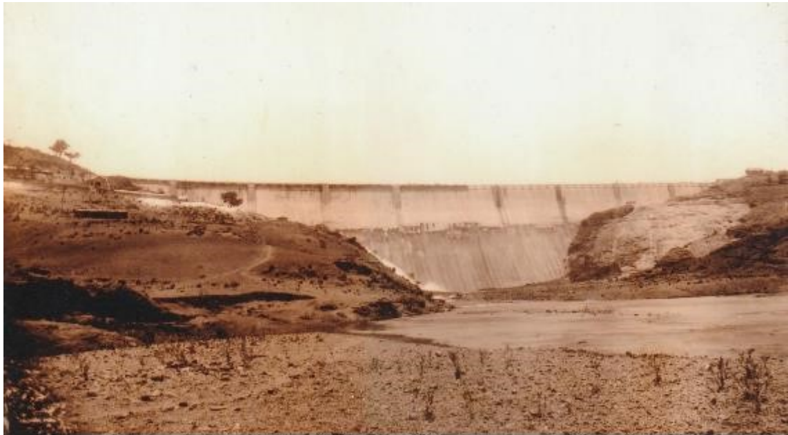
22 - Dam At the End of May 1924 , Height 270 Ft, Above River Bed, Down Stream View
