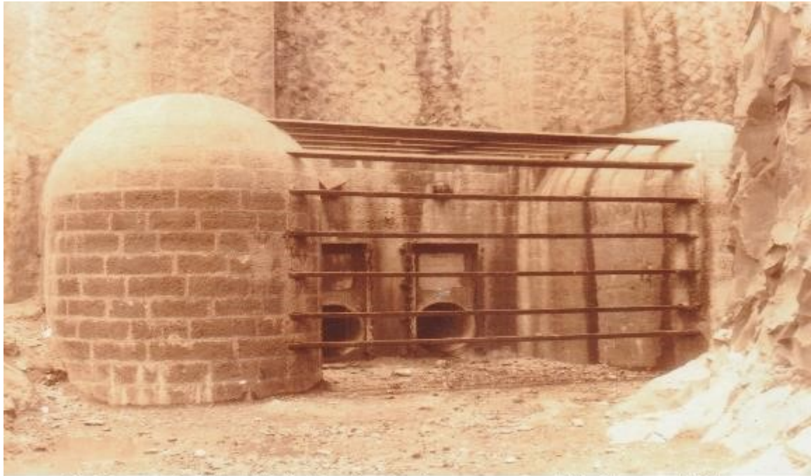
72 - Lowest Outlet at 50 Ft. Showing Caging arrangement Up Stream - 1919
