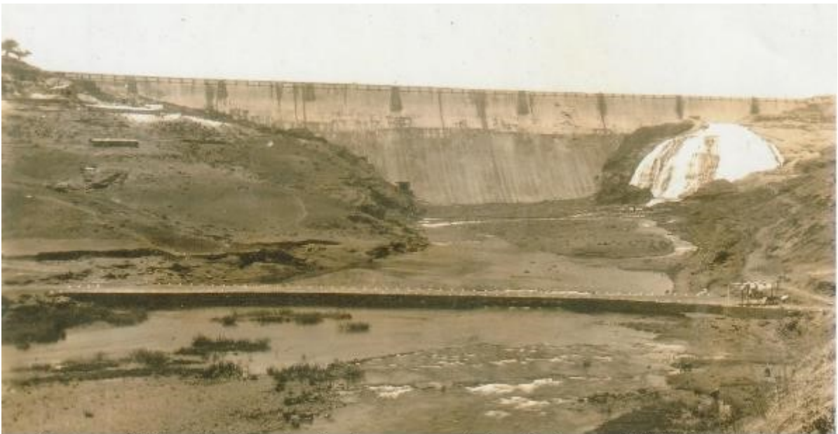
40 - General View of the Dam showing the cause way below the Dam and 200 Ft. Sluice Open
