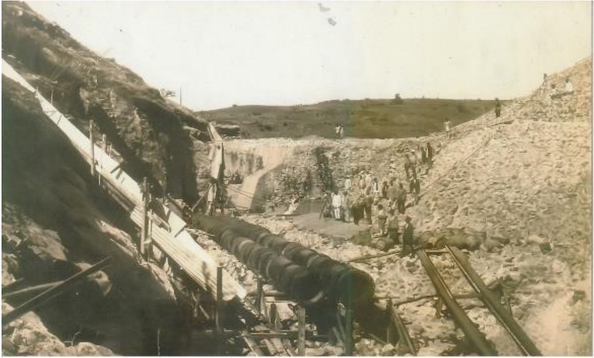
Photograph of installing A 50 foot Vault in the Wall.
