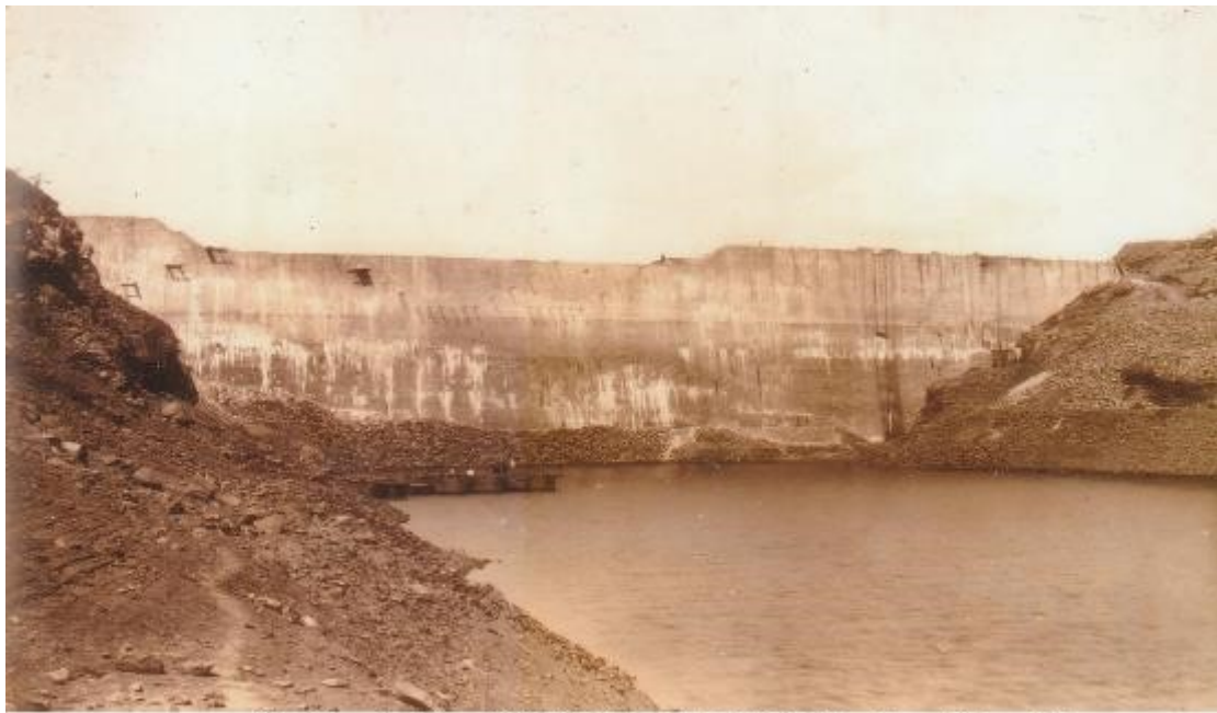
67 - Dam in May 1919 Effective Height 155 Ft. Above River Bed Up Stream face from the North Bank.
