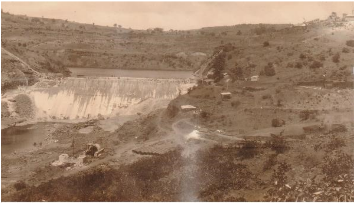
12 - Lake- Arthur Hill Dam - Full View of the Dam 85 Ft high taken from the Left Bank ( June - 1915)
